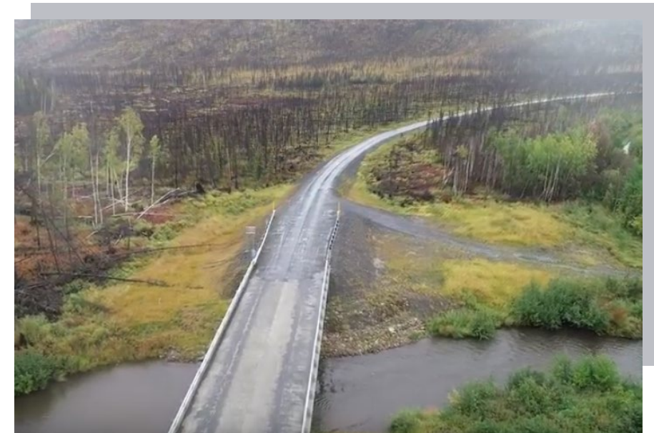
Completed bridge over Boulder Creek
