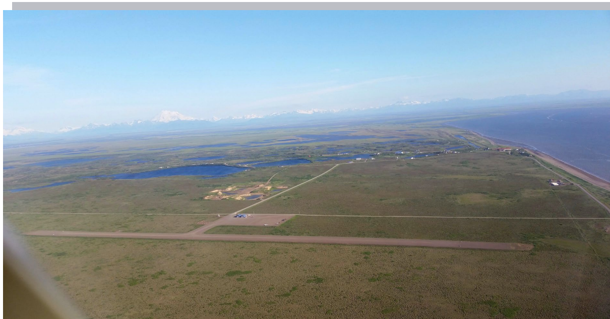
Existing Pilot Point runway Photo credit: Alaska DOT&PF
