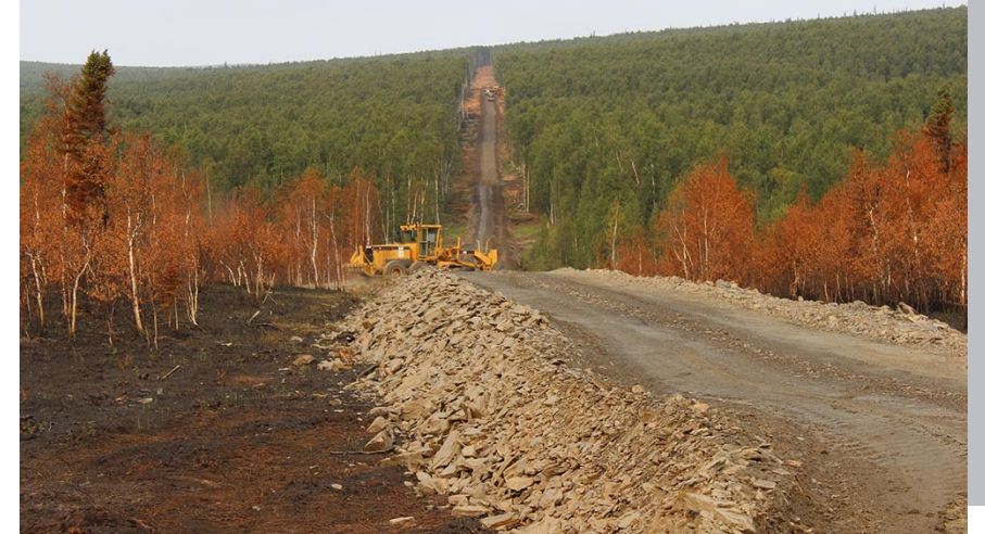
Construction ongoing in August 2015
