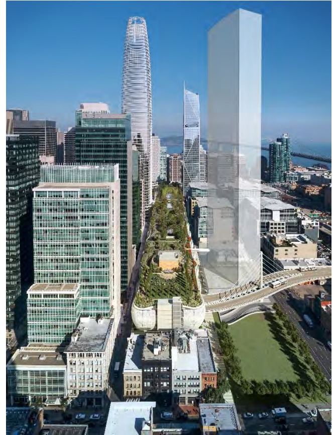
Transbay Transit Center, San Francisco, CA
