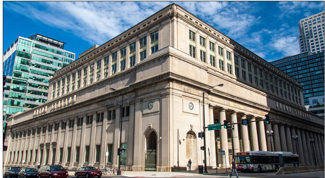
Headhouse Building on Corner of Jackson Blvd. and Canal St.
